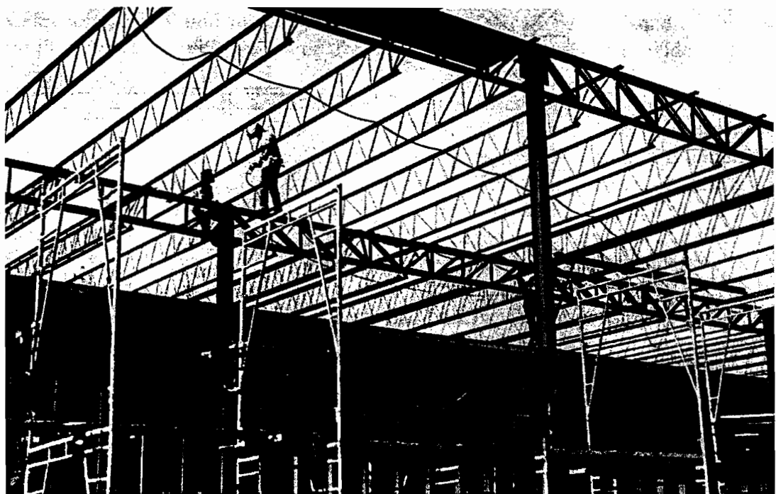
PHOTO 9-1 Typical roof and deck construction for a two-story office building. Open web steel joists for the roof are being welded to supporting joist girders.
