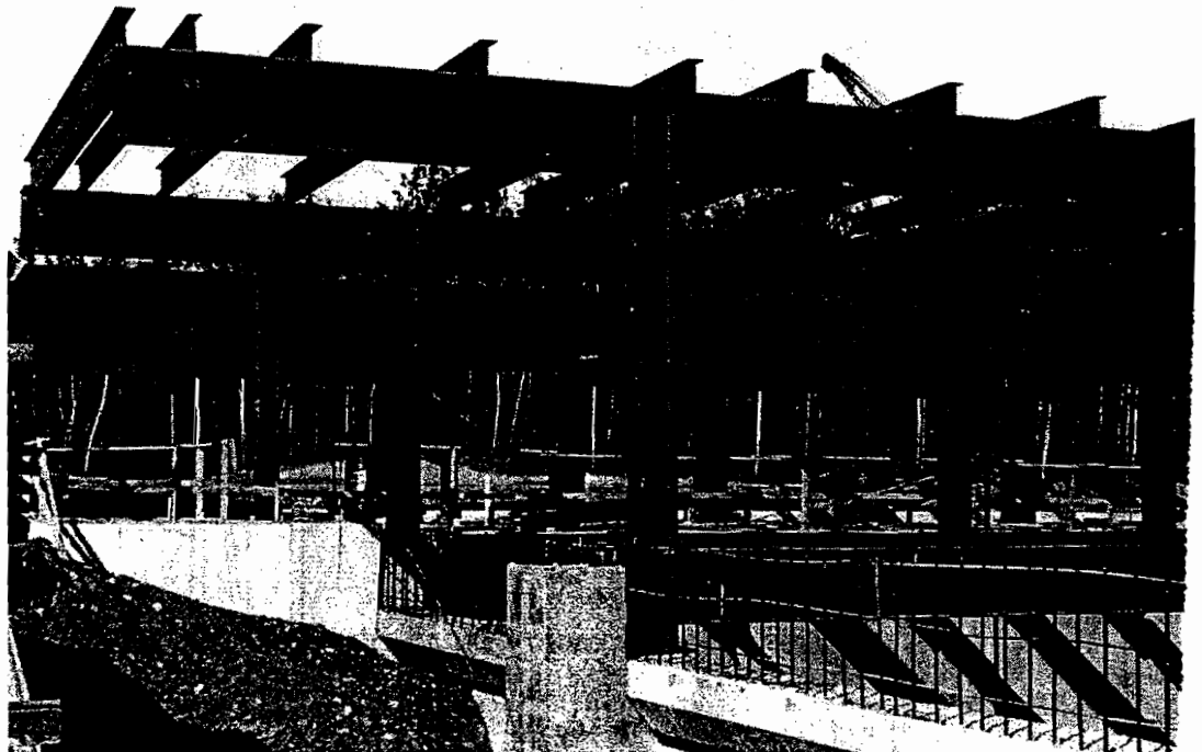
PHOTO 4-1 Overhanging beams. Note the bearing plates and web stiffeners at the supports.
