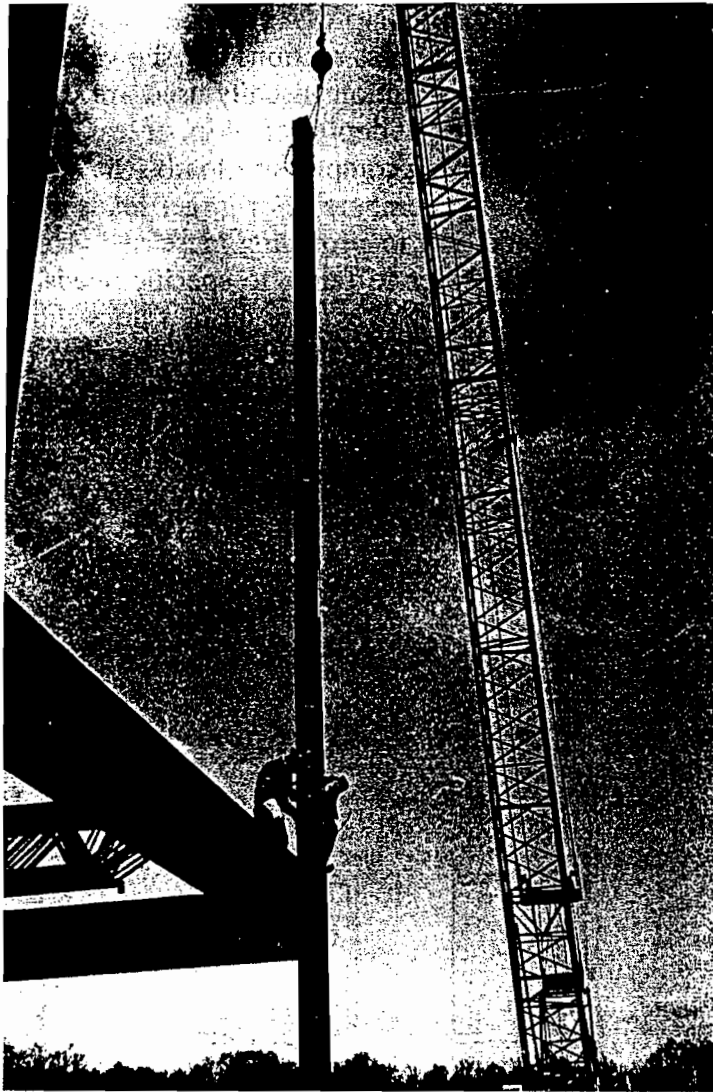
PHOTO 3-1 Erecting a three-story structural steel wide-flange column.
