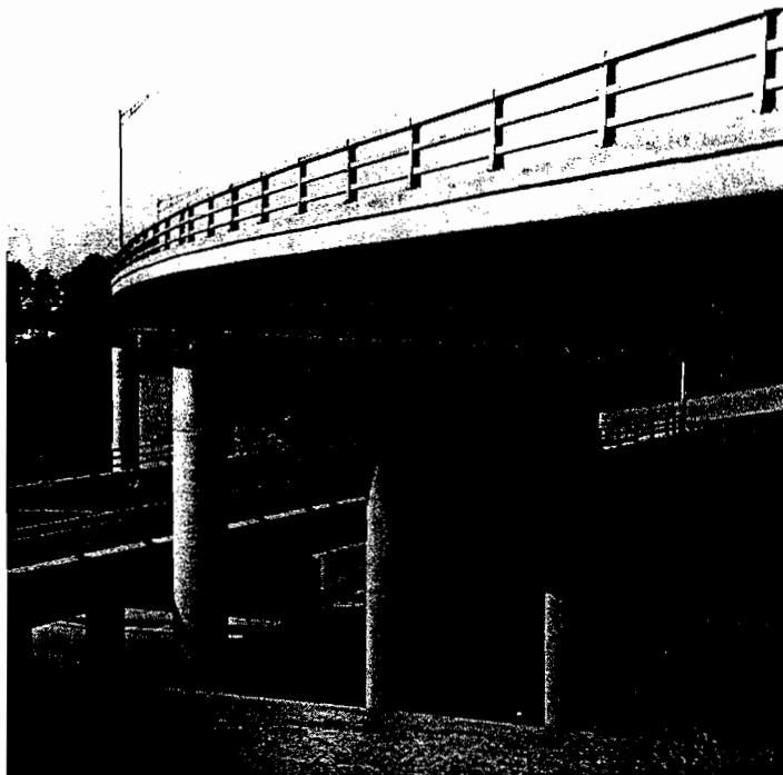
PHOTO 5-1 Plate girder highway grade separation bridge near Rochester, New York. Girders are simple spans and carry a curved upper roadway. Note variable-thickness bottom flange and intermediate transverse stiffeners. (Courtesy of the New York State Department of Transportation.)
